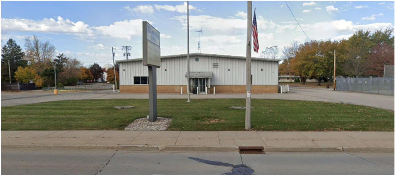
Richmond Hall existing condition
