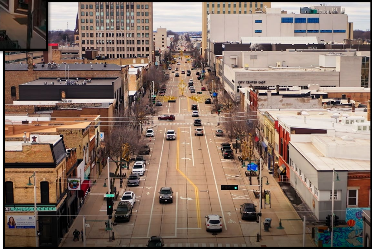
Figure 13: College Avenue Road Diet A road diet on College Avenue would reduce the number of through lanes in each direction to provide room for a center two-way left turn lane and bike lanes. AECOM
