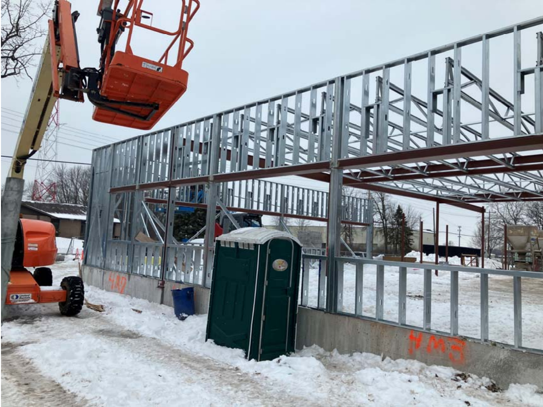
Figure 2: Valley Transit Whitman Ave facility renovation progress.
