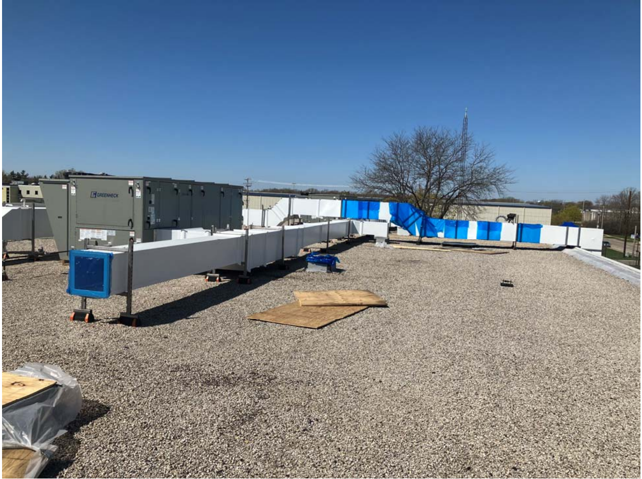
Figure 4: Municipal Services Building mechanic shop HVAC upgrades.
