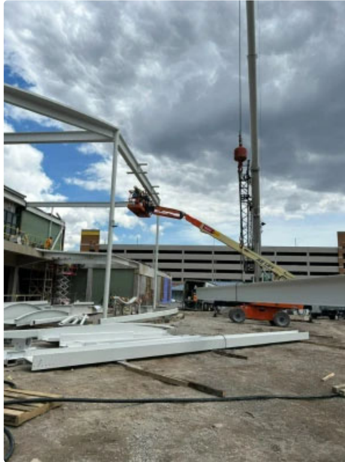
Front exterior steel installation - "The Commons"
