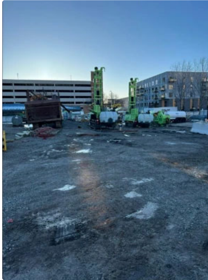
Geothermal well drilling
