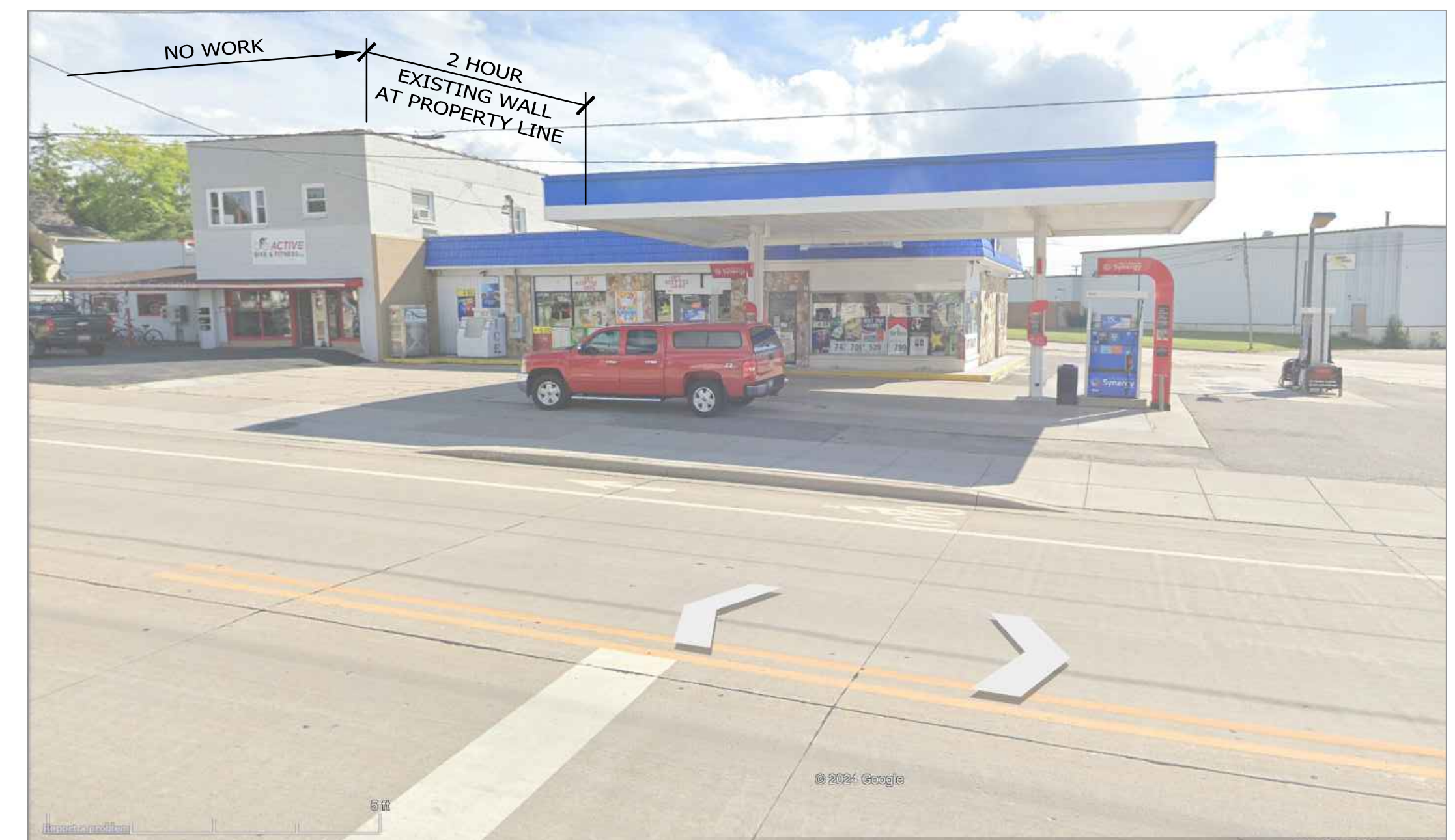
REFERENCE PHOTO AT BADGER AVE SCALE: NO SCALE (FRONT) 1 A3.1
