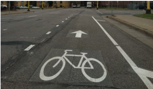
Recessed thermoplastic bike lane symbol. Alta.
