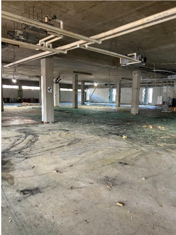
Northeast Ground Level
