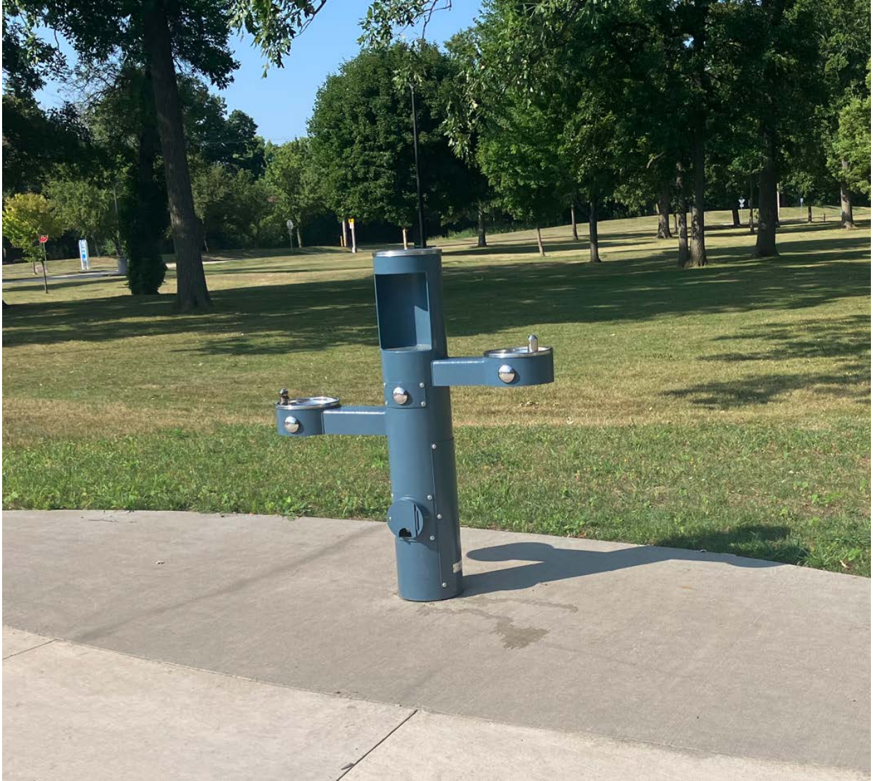
Figure 7: Telulah Park drinking fountain installed.
