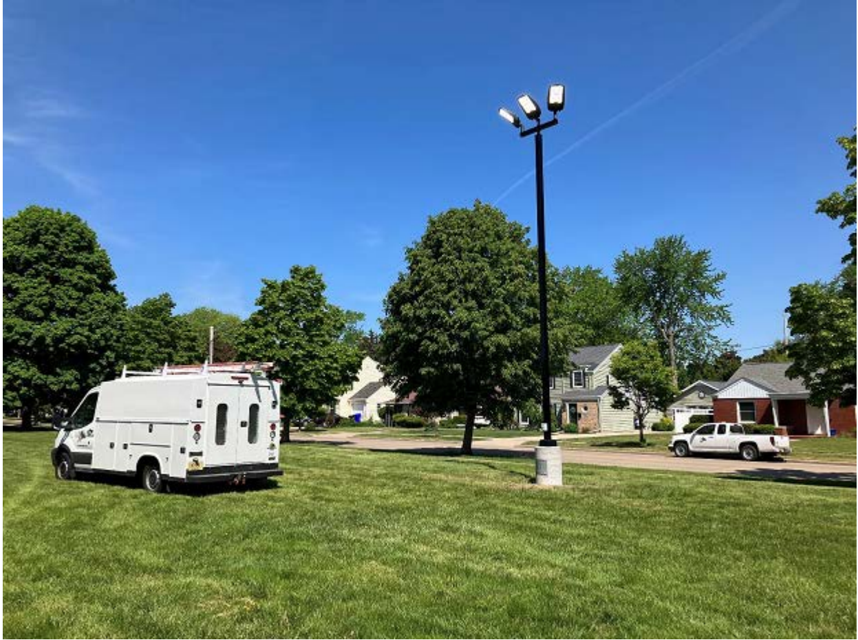
Figure 4: Erb Park site light installed.
