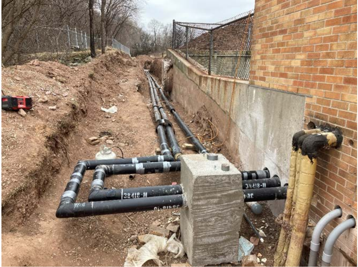
Figure 14: Wastewater Treatment Plant HVAC upgrades for H & J buildings.
