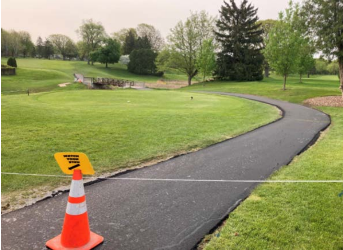
Figure 10: Reid Golf Course cart path paving.
