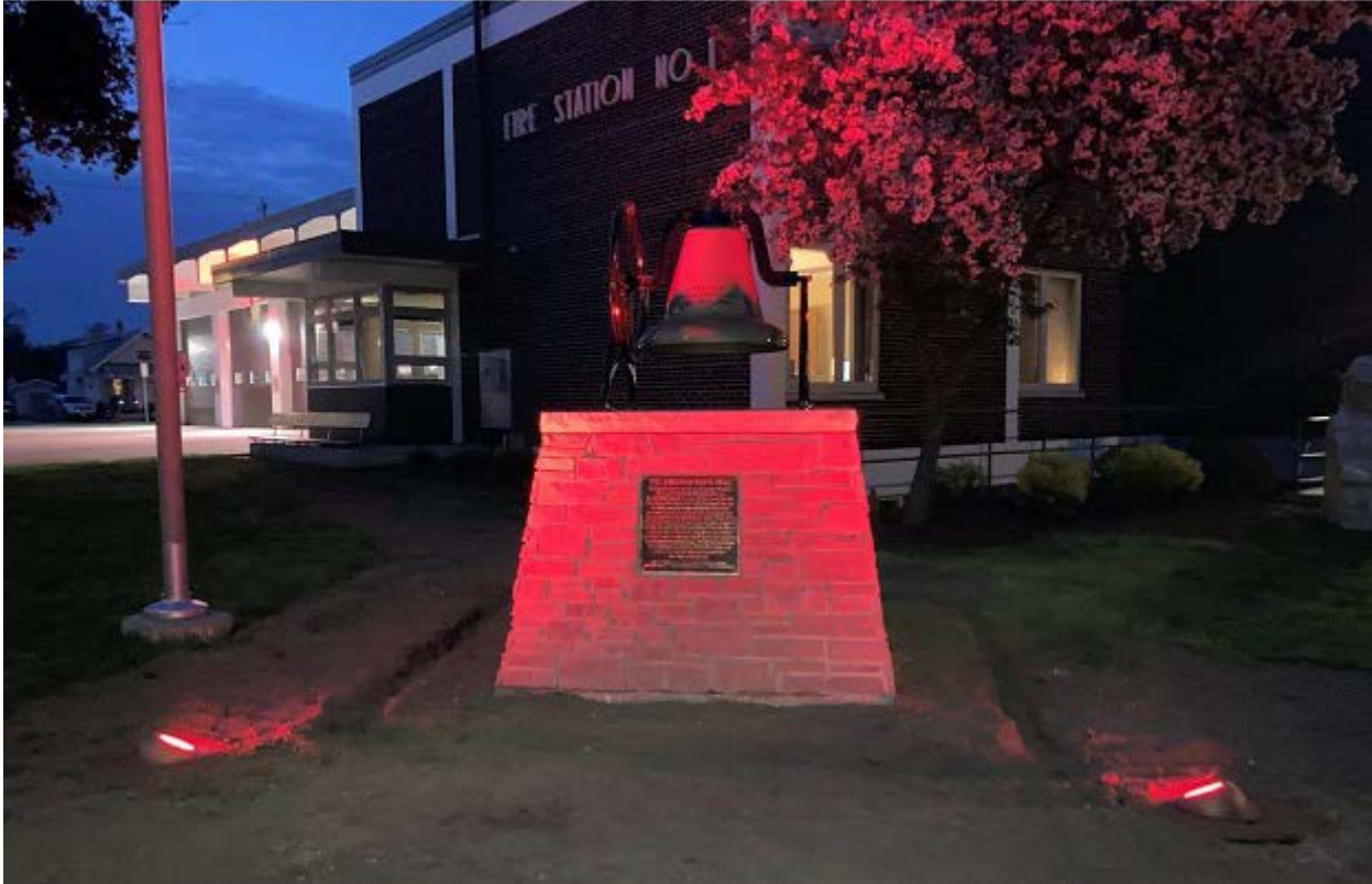
Figure 5: Fire Station #1 bell tower lighting installed.
