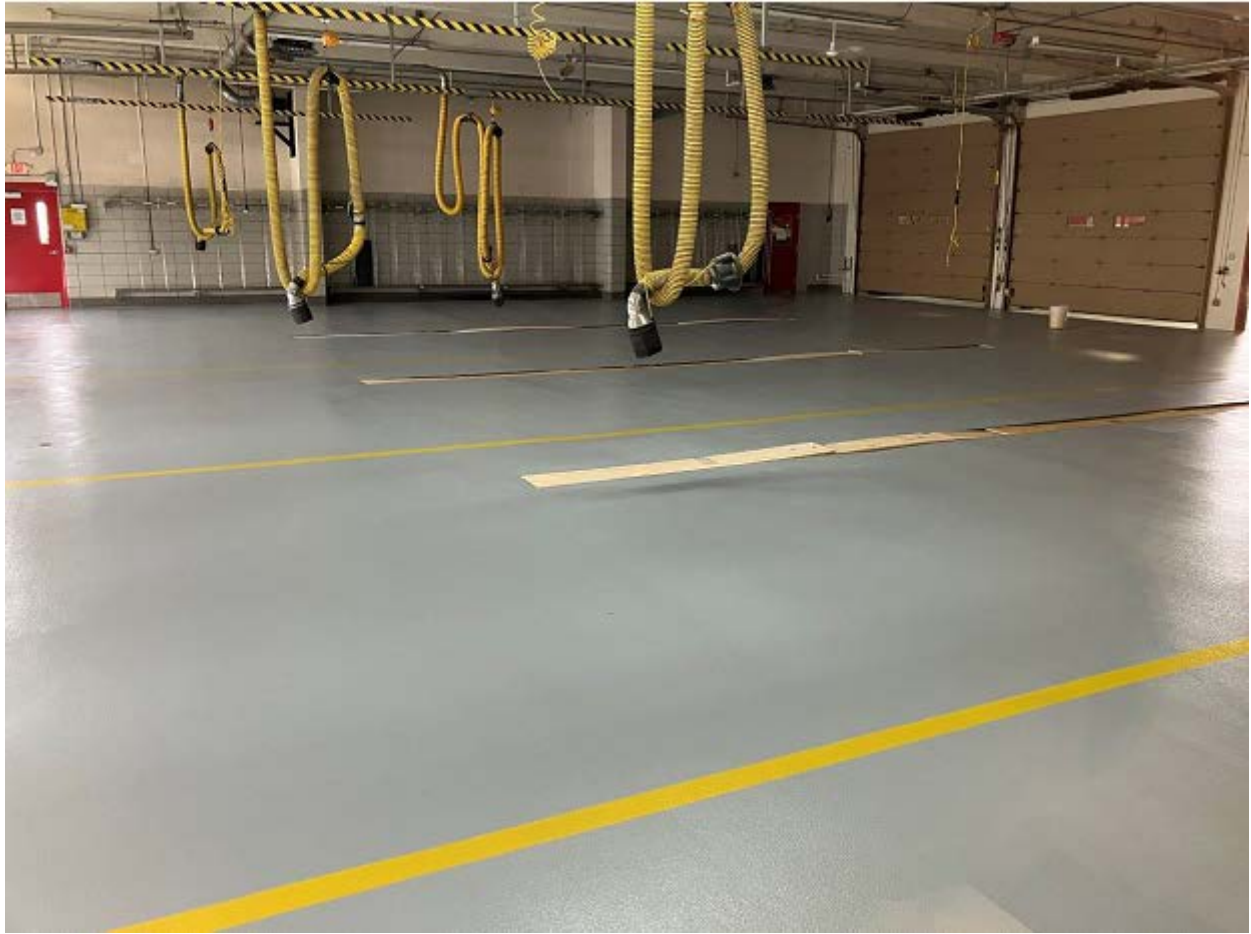
Figure 3: Fire Station #1 rig room floor epoxy replacement
