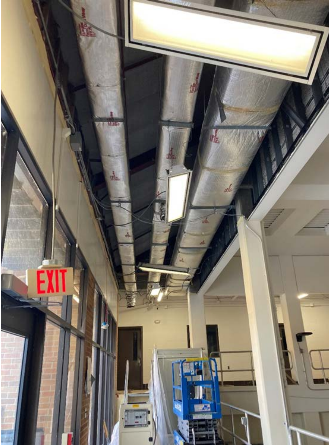
Figure 13: Wastewater Treatment Plant V-building painting.
