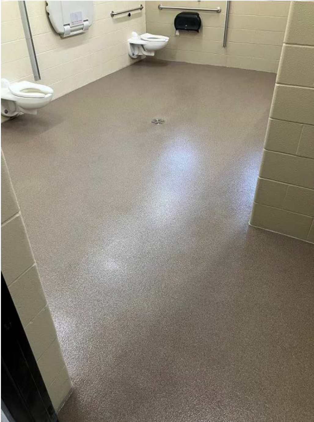
Figure 2: Jones Park pavilion restroom epoxy floor coating installed.
