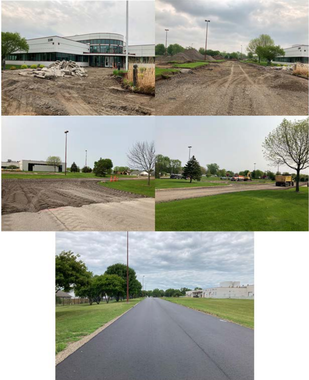
Figure 11: Water Treatment Plant hardscape replacement.
