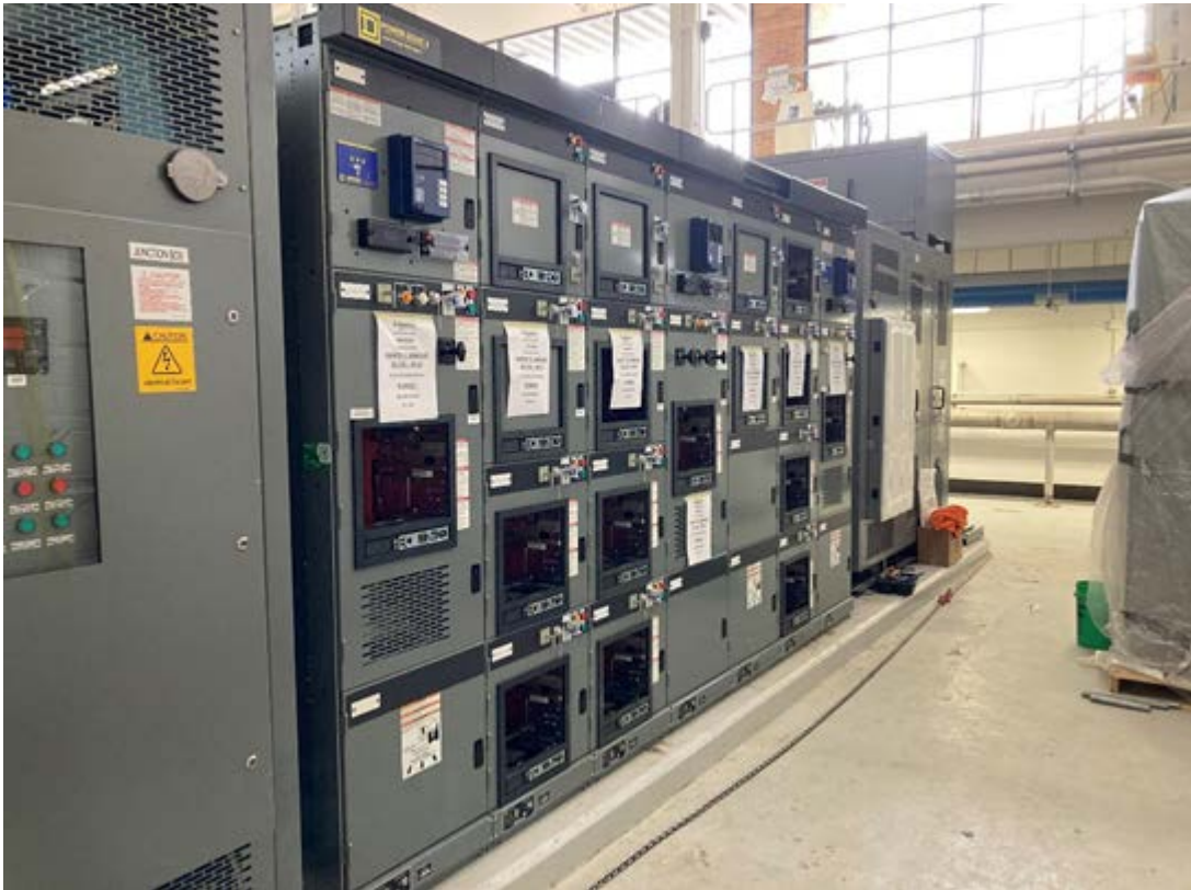
Figure 12: Wastewater Treatment Plant electrical distribution upgrades.
