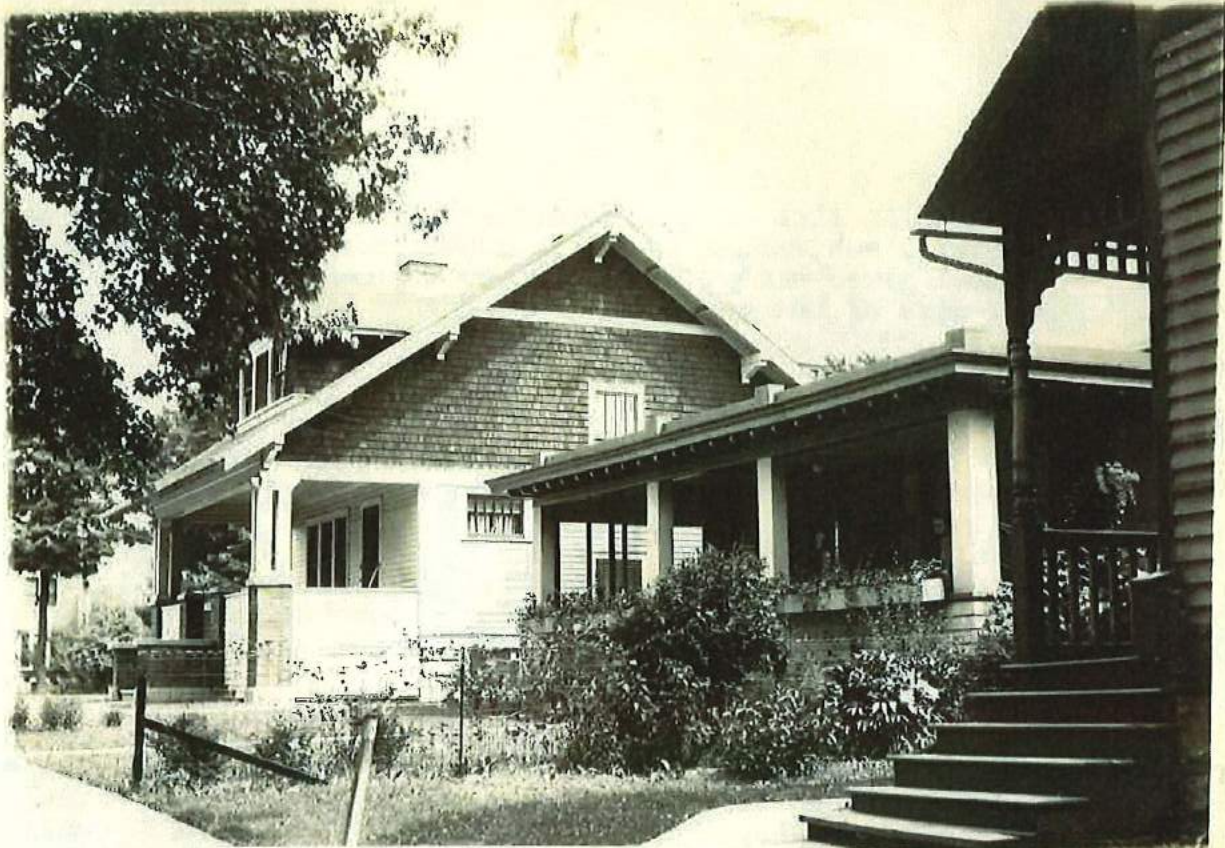
photo #21. Lack of building line on sixth street.
