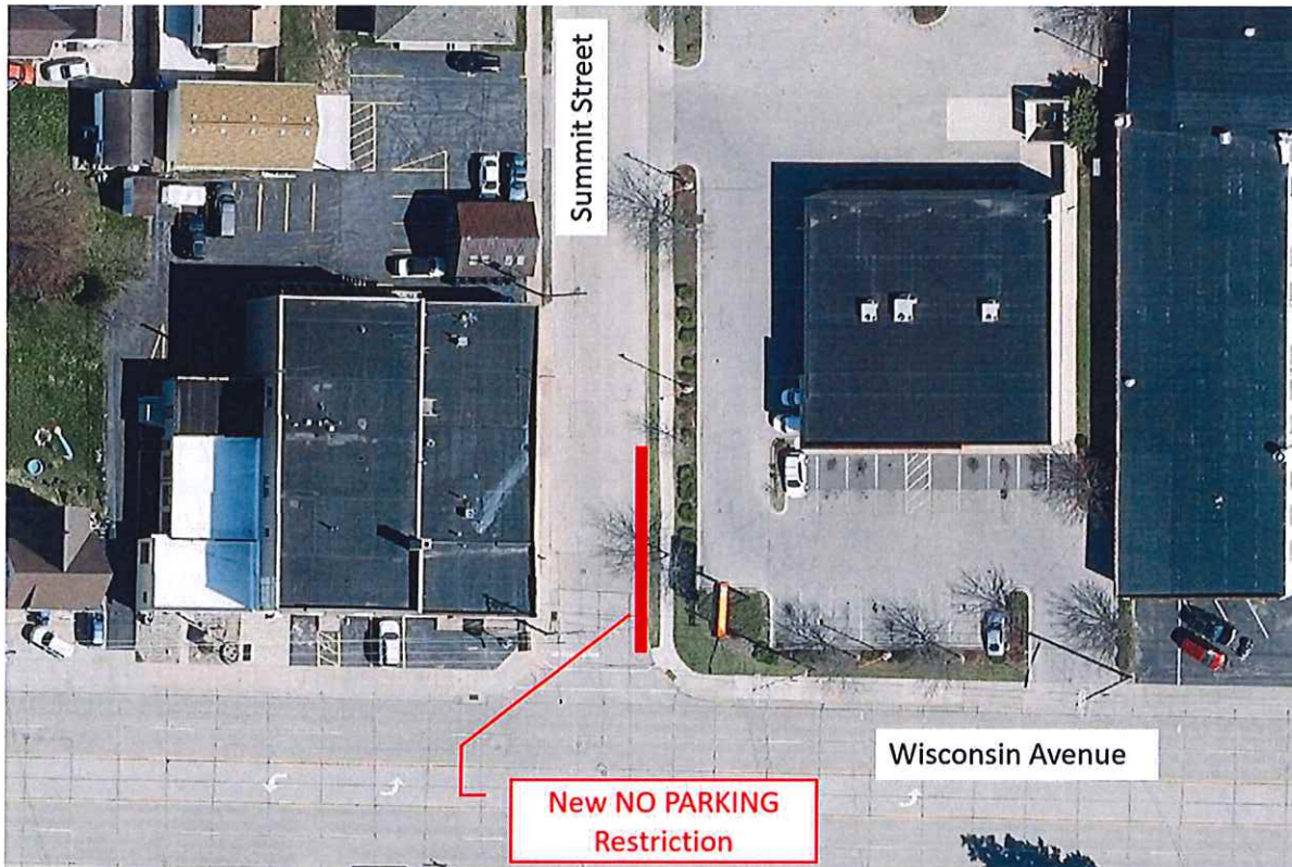
Figure 1: New NO PARKING Restriction, east side of Summit Street, extending 75-FT north of Wisconsin Avenue
