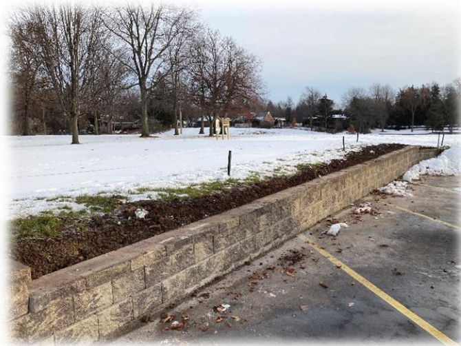
Retaining wall completed and backfilled.
