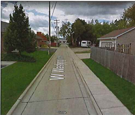
Figure 1- 800 W. Washington St (looking west)
