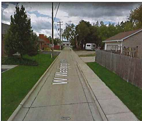
Figure 1- 800 W. Washington St (looking west)
