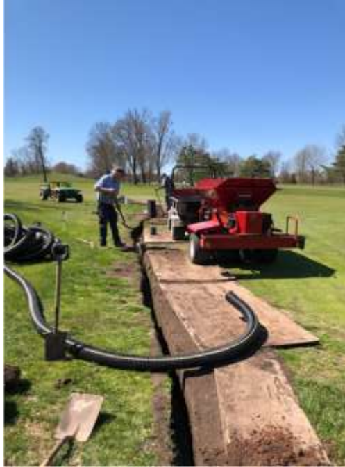
Staff working on drain tile on #14.
