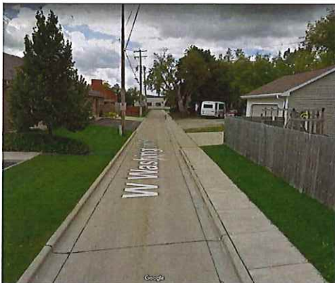
Figure 1- 800 W. Washington St (looking west)
