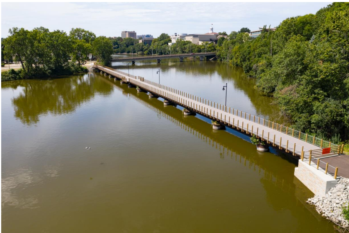
Lawe Street Trestle Conversion - 2020
